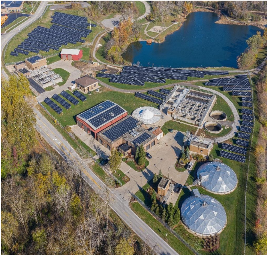
Water Treatment Facility City of Plano, Illinois Annual Production = 1.3 million kWh/year Lifetime Production = 32.5 million kwh's
