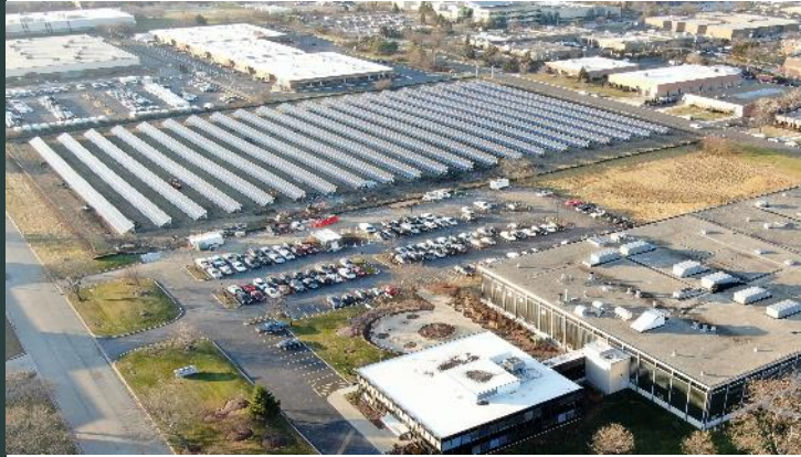
Toyoda Amercias Arlington Heights, IL System Size – 1.66 MW 5,040 modules
